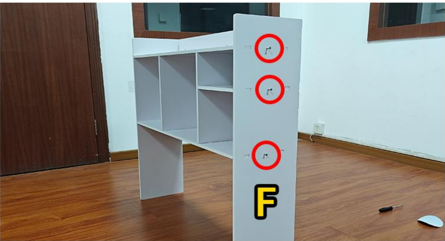
10.AS SHOWN IN THE FIGURE; FIX THE SCREWS, THERE ARE A TOTAL OF EIGHTEEN
