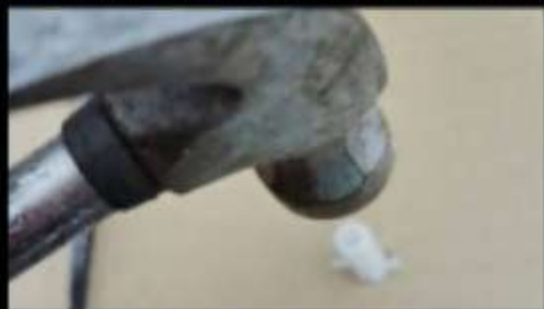
5.将涨塞打入墙体 DRIVE THE EXPANSION PLUG INTO THE WALL
