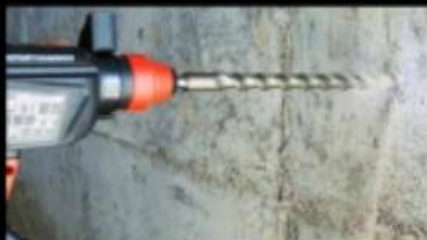
4.冲击钻打孔 PERCUSSION DRILLING
