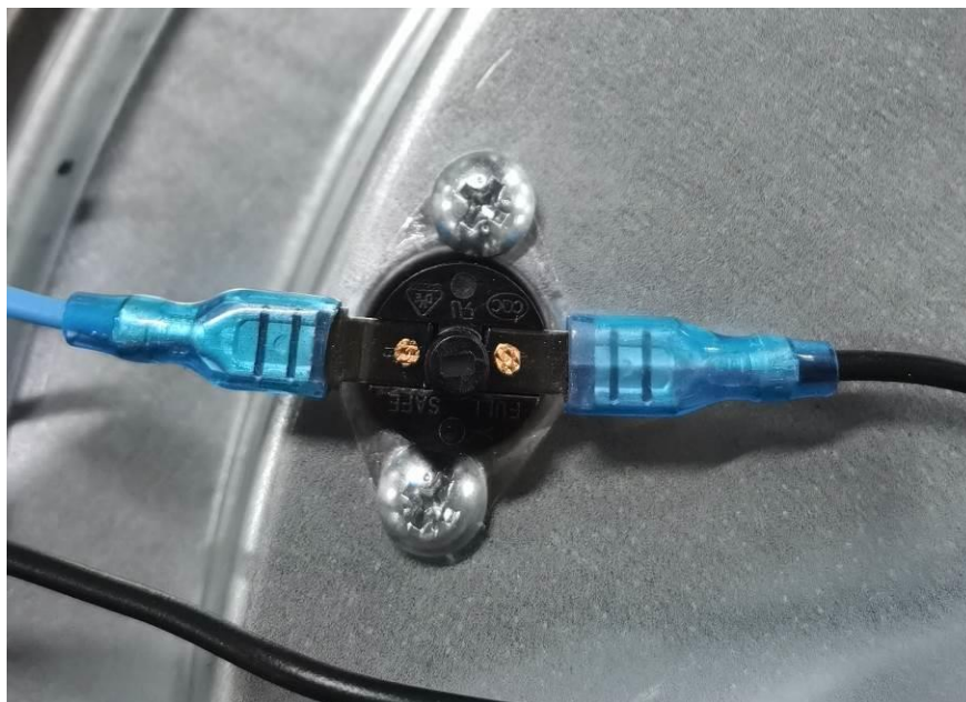
Non-self-reset Thermal Cut-out
