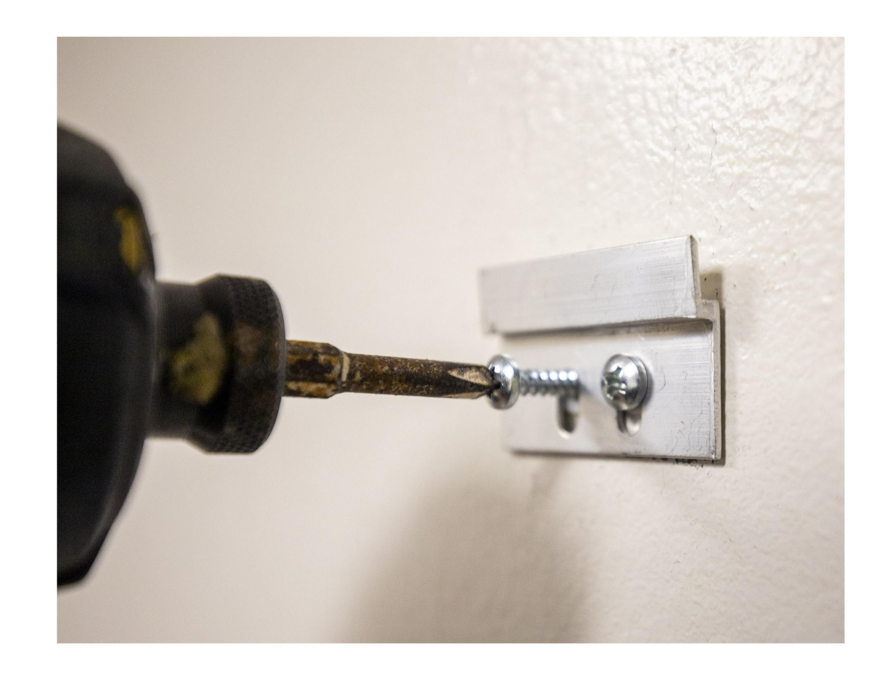
Step 9: Using a drill with a phillips head bit and the screws provided, fasten the cleat to the wall. (repeat for the other side)
