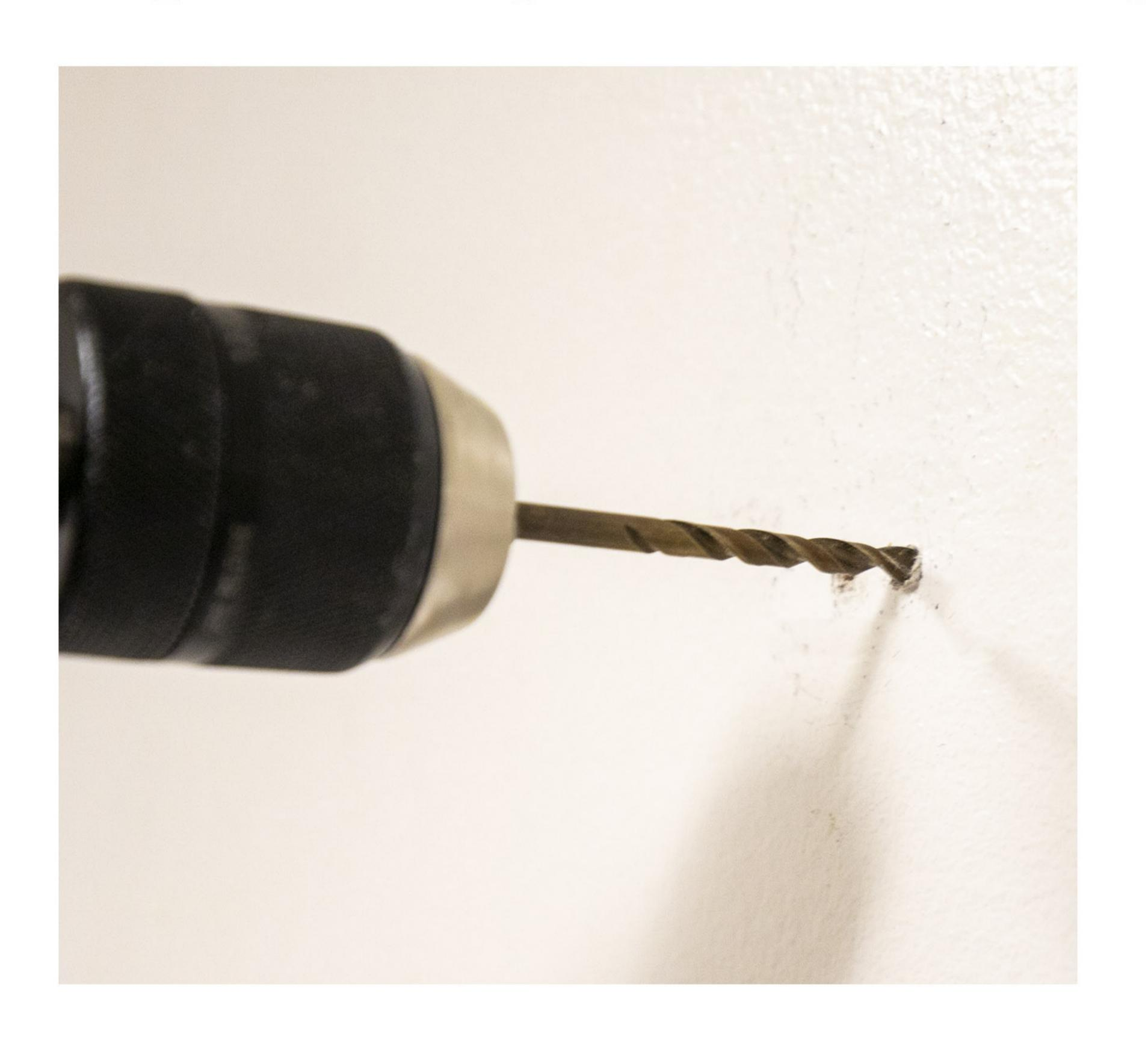
Step 7: Using a drill and 3/16" bit, drill holes where you marked in step 5.
