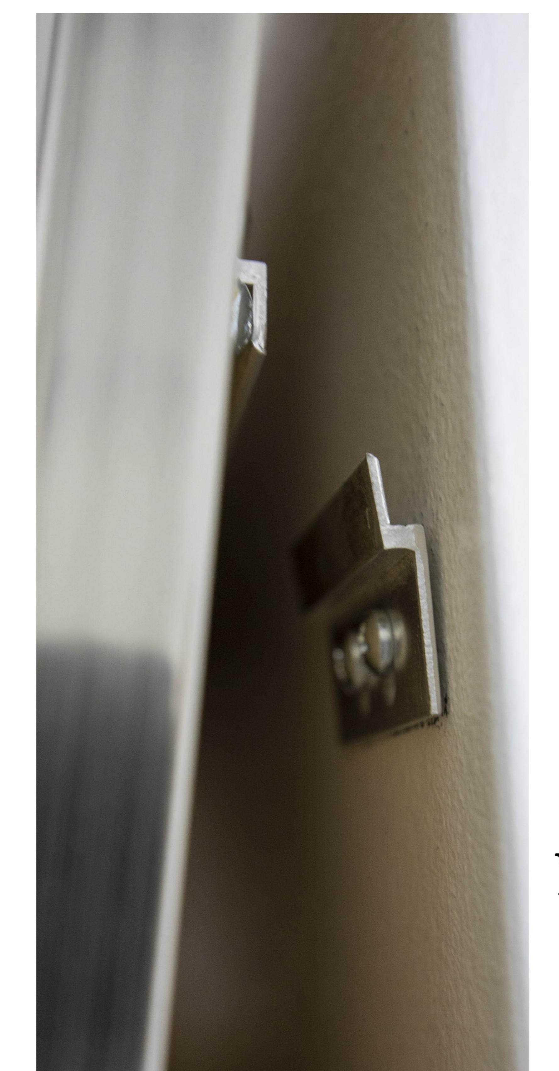
Lift your mirror so the cleats are slightly above the ones on the wall and set it down.
