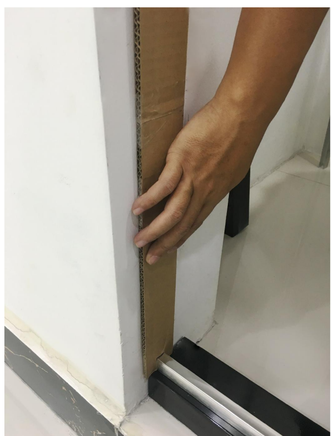
Insert template to bottom door guide.
