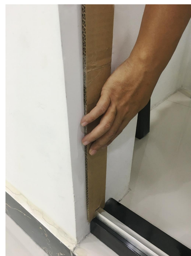
Insert template to bottom door guide.
