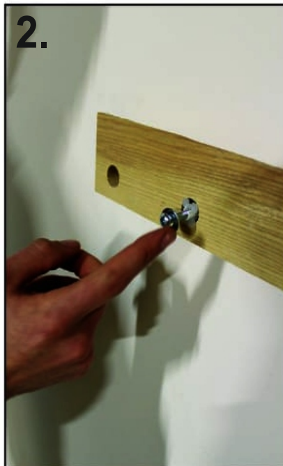
2. Thread the metal screw through the plastic washer until it threads till the wall
