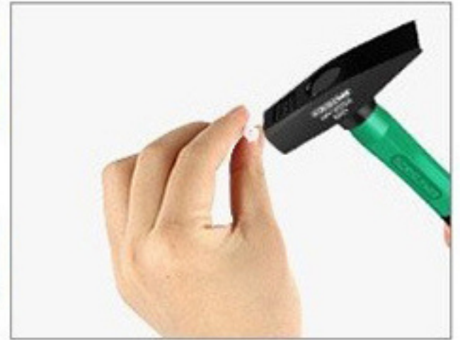
3. Drive the expansion screw into the wall
