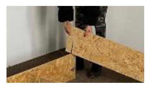
3. Stand the other **Side Piece** up on its side with the slit opening facing <u>UP</u>. Align the **Side Piece** with the other end of the **Head Piece** and slip the **Head Piece** into the opening of the **Side Piece**. Ensure the two pieces are secured together by pushing the **Head Piece** all the way down.
