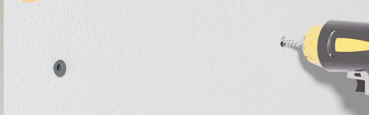
04 Drill holes in the wall
