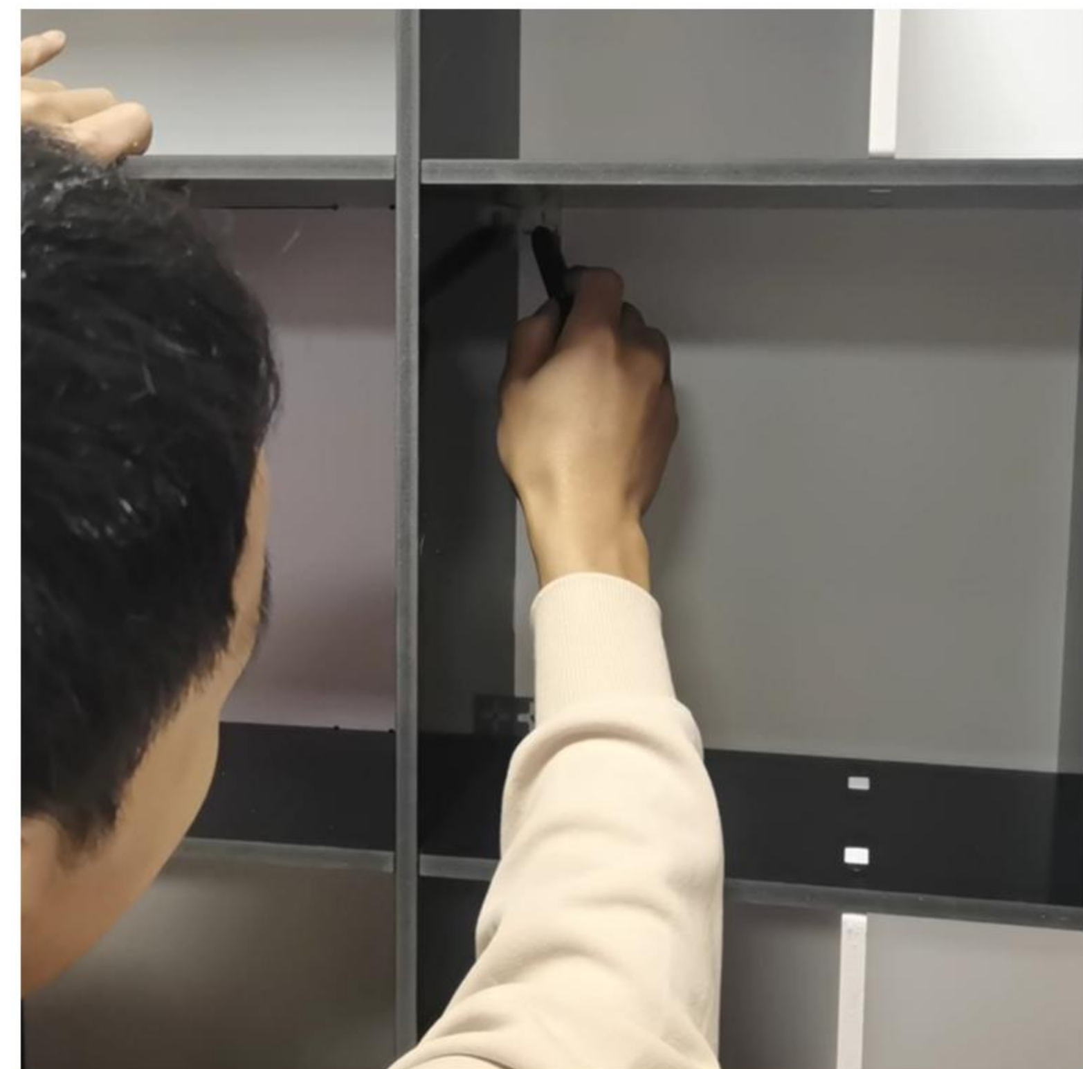
1. MARK THE HOLE WITH A MARKER
