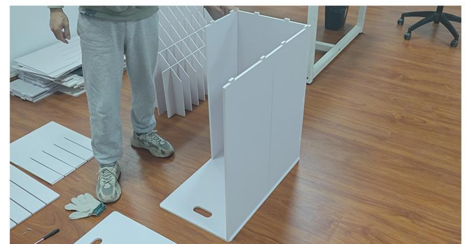
8. THE UPPER I PLATE IS ASSEMBLED WITH THE J PLATE
