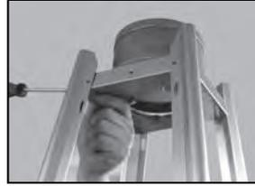
**STEP 7:** Take out 3 two sided bolts (Part A) out of screw pack, and connect to flame screen(Part AA). Attach reflector(Part G) through the 3 bolts. Then tighten the shield with the 3 wing nuts.
