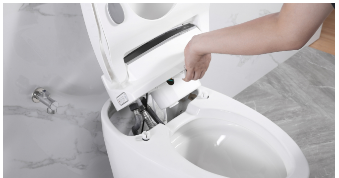
Step 1. Cut off the power supply and lift the toilet seat forcefully upwards
