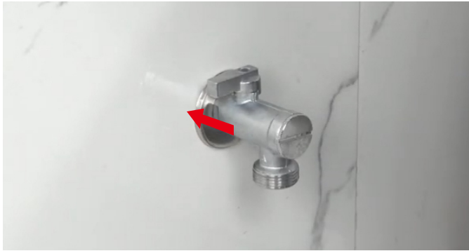
17. Fix the Angle valve to the wall.
