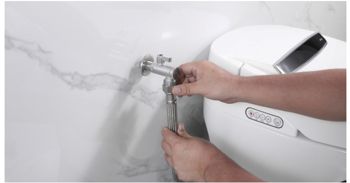
18. Finally connecting the flexible tube to the inlet angle valve.
