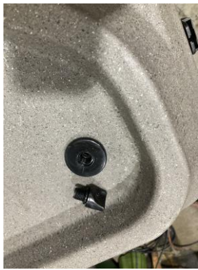
Air bleed valve opened
