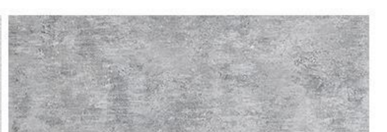
Concrete wall surface
