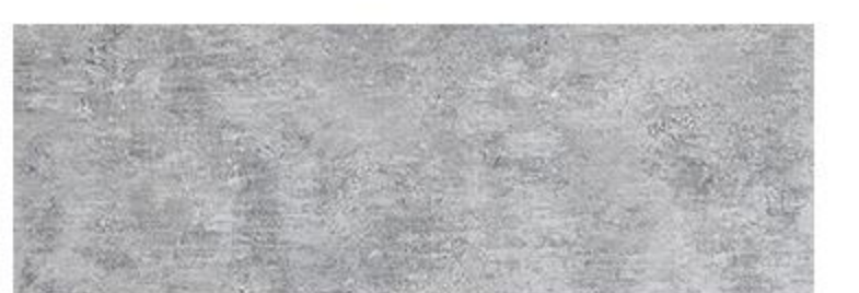
Concrete wall surface
