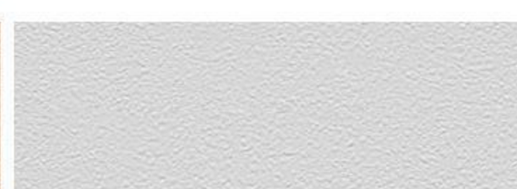
Latex paint wall
