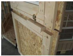
Barrel bolt is installed and 3/16" hole is drilled. This is what it looks like when completed.
