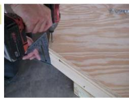
Next secure plywood to joint and rim as shown using 1 1/4" Zinc Screws.
