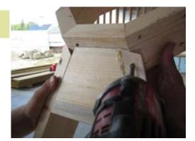
Install first rafter to Octagon as shown at pencil marked as shown.
