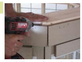
Insert 2 1/2" screws in an angle to tie top plates together.
