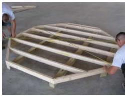
Secure all corners of 4x4s with 2 1/2" Screws. Next measure floor for square as shown.
