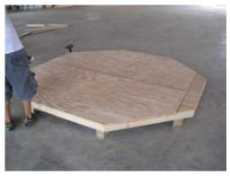
The plywood is all cut. You may have to lay the flooring out before you fasten anything to make sure the pieces are placed properly.
