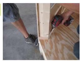
Secure wall panel A with 2 1/2" screws as shown. make sure corners line up and put pressure on the outside pushing in so wall is tight against floor as shown.
