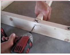
The rims are also marked off where the joist need to go. Secure joist with 2 1/2" Zinc screws.
