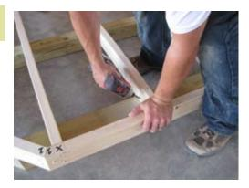
Once floor is square secure all the joist to the 4x4 runners as shown. Angle 2 1/2" screws thru joist into 4x4 runner. One on each side.
