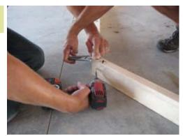
Next secure rim with 2 1/2" Zinc screws as shown. Make sure all points are flush as shown.
