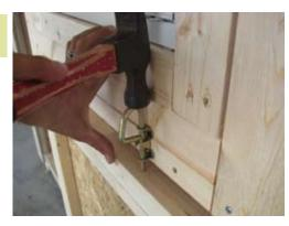
Secure with 1 1/4" screws. Use hammer and tap on top of bolt as shown to locate hole to drill.
