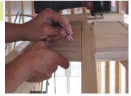
Secure blocks with 2 1/2" screws as shown.
