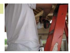
Push metal corner up until it is against top and secure with 1 1/4" Zinc Screws.
