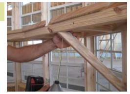
If wood wants to split use 1/8" drill bit and drill hole where screw is shown to go through.
