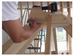
After all rafters are installed and fastened, fill in blocks that are cut on angles in between rafters.
