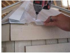
Secure with 1" white screws with rubber washer.
