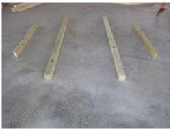
Locate 4x4 runners for 8x8 Octagon Greenhouse. Layout 4x4's as shown.
