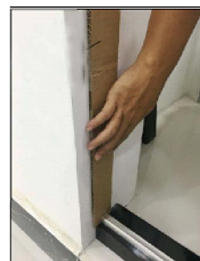
Insert template to bottom door guide.
