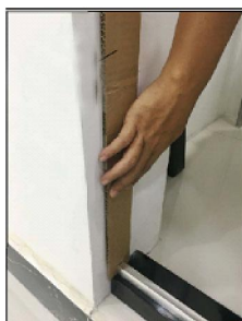
Insert template to bottom door guide.
