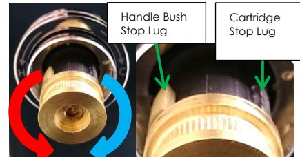
5. Now re-fit the Handle Bush so that the Stop Lug is not in contact with the Cartridge Stop Lug and rotate the Handle Bush fully clockwise until a 'click' is heard. Should the Stop Lugs come into contact before the click, simply remove the Handle Bush, turn it half a turn anti-clockwise, fit it back onto the cartridge and continue to rotate it clockwise. Repeat this process until you hear the click.
