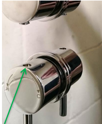
1. Remove the Temperature Handle concealing cap.
