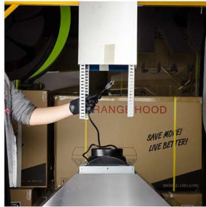
18. Connect the duct to the damper/air flapper onto the main unit.
