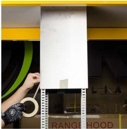
17. As pictured, each corner uses 4 screws to secure the main unit to the support frame.
