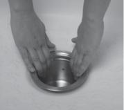
2). Screw in the Drain (F) to secure it to the tub.
