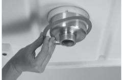
3). Underneath the base of the tub, place the Washer (I) over the bottom of the Drain (F).
