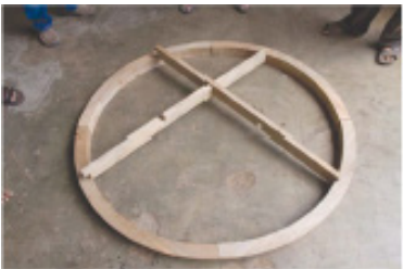
Cross beams for the top are added.
