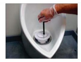
2. Pull upward on insert to remove.
