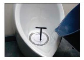
1. Using the key provided, screw the key into the key hole of the drain insert and fill with water.
