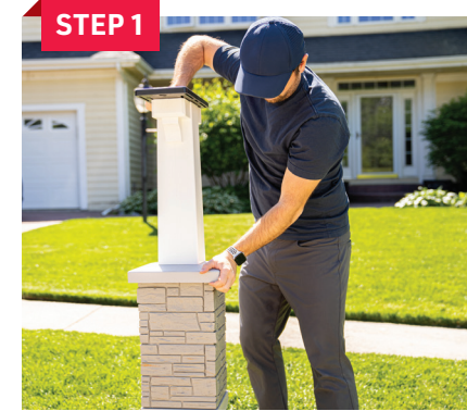
STEP 1 Install mailbox post over 4x4 until flush with the ground surface.
