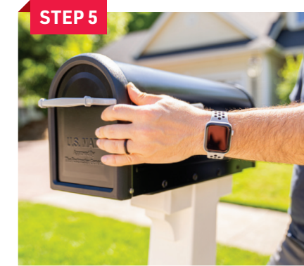
STEP 5 Place mailbox over the mounting plate and slide forward or back to desired position.
