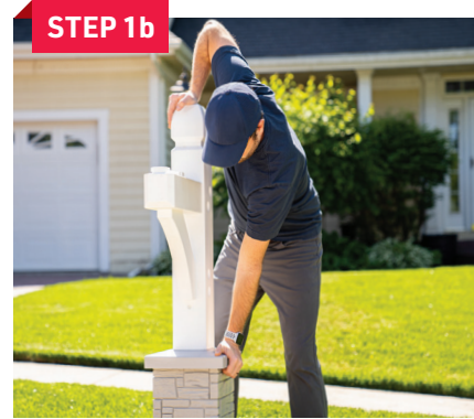
STEP 1b Push the post downward until flush with the ground surface.
