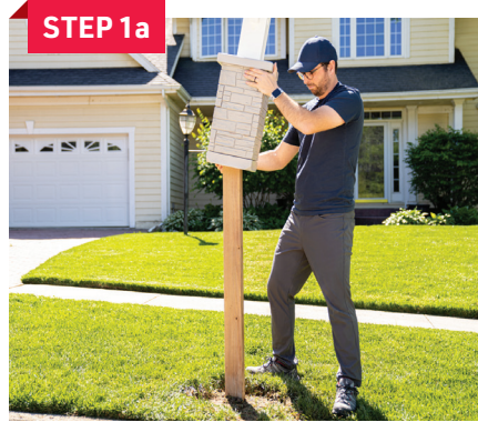
STEP 1a Install post assembly over 4x4. Ensure front of mailbox will face the street correctly.
