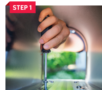
STEP 1 To remove or replace an installed mailbox, the screws need to be removed to lift off the mailbox.
