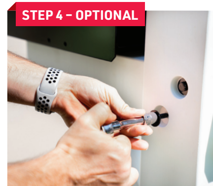
STEP 4 - OPTIONAL Cross-arm model only. Pre-drill the center of four inset holes on the side of post (eight total). Use a 1/2" socket to tighten the lag screws and washers into position.
