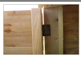
Align the top hinge in place, ensuring that the gap between the door and post is consistent at top and bottom.
