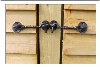
To fit the latch keeper plates, shut the door and hold the latch in the horizontal position. Now fit the keeper and mark its correct fixing position on the centre post using a pencil or bradawl before securing it in place using the screws provided.
