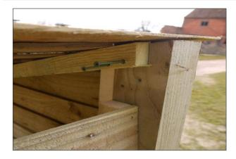
Secure the rear of the roof using shorter green screws as shown.
