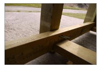
Check the positioning of the post within the guide marks once again before securing the bottom of the centre post with 2 of the longer green screws
