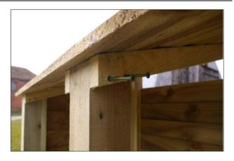
With the centre post now attached to the base, locate the top of the post between the central roof battens, flush with the batten ends, and secure in place with 2 of the shorter green screws.
