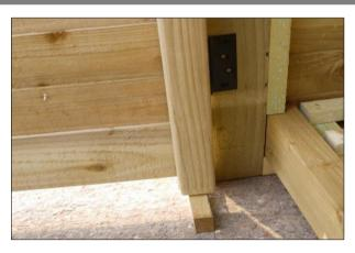
Place a spacer block at the front of the log store adjacent to the front end post and rest the hinge side of the appropriate door on the block, aligning it vertically and horizontally for a good fit. Now use four of the supplied black hinge screws to affix the hinge to the post.
