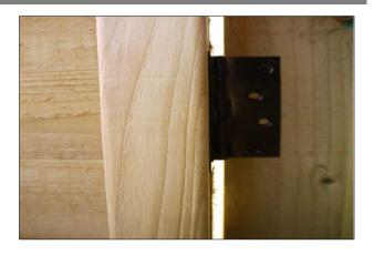
Secure the top hinge in place using more of the black hinge screws. Repeat steps 19 - 21 for any further doors as required.
