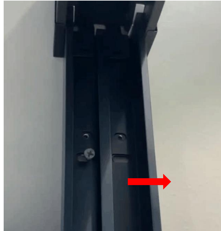
Loose the diagonal line profile screws to move outside shower direction.
