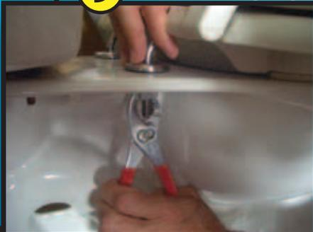
Secure the seat using pliers...
