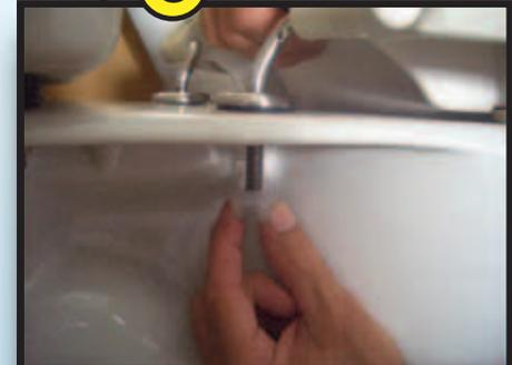
Finger tighten the nuts...make sure that the seat is mounted properly
