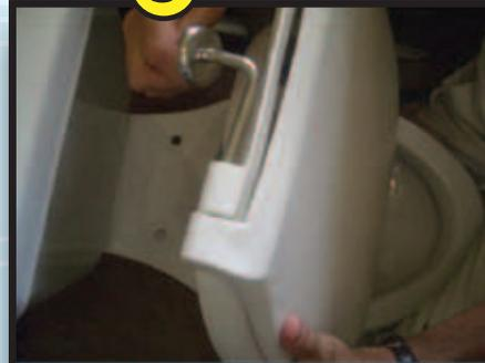
Insert the Left Hinge through the seat and lid on the Left side\*
