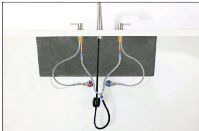
6. The installation is complete. You can open the handle and check whether there's leaking or not.
