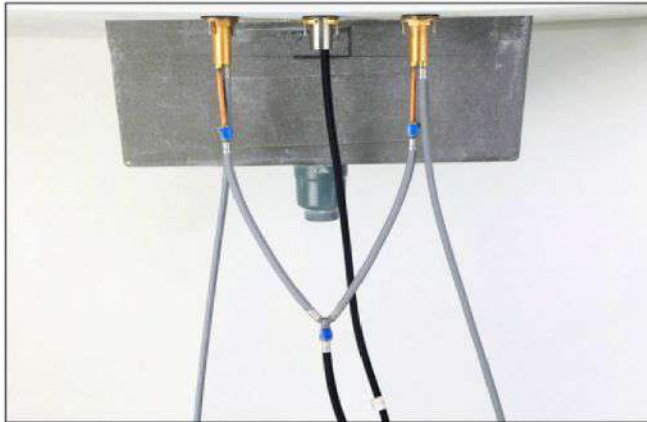
3. V shape hose connection. Make the black hose, two brass hoses connect to the V shape hose.
