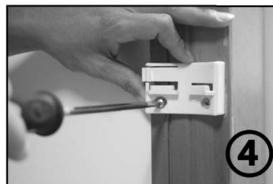
Fix A1 & A2 with screws on the surface firmly.
