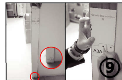
Put Scale Direction R on the desired location, make sure the bottom of A4 is 28mm to the floor and mark the screw holes of A3 & A4 on the surface.
