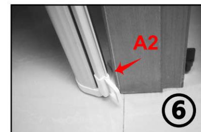
Install and fix the metal tube on A2 & A1.
