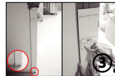
Put Scale Direction L on the desired location, make sure to suck the bottom line of A2 to the floor and mark the screw holes of A1 & A2 on the surface.
