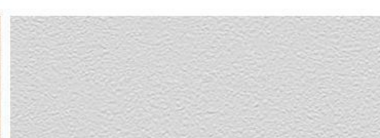
Latex paint wall
