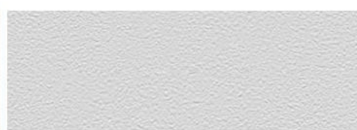
Latex paint wall
