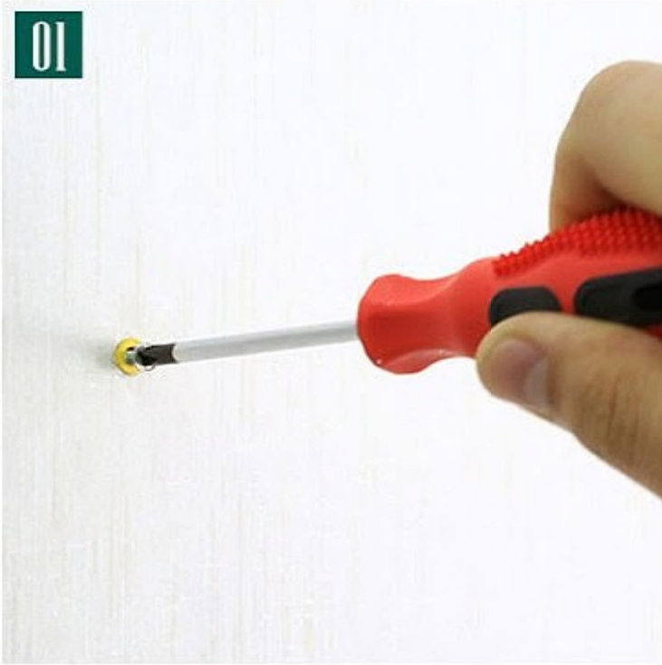
Install the expansion screw into the wall
