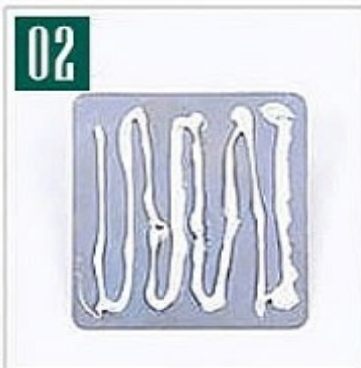
Apply a sufficient amount of nail free adhesive evenly on
