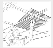
2. For edge trim pieces that need to be cut, measure for the dimensions needed and cut with a circular saw.
